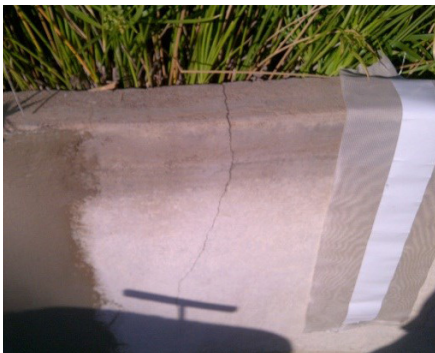
Photo 4: Typical crack in a reservoir structure SEALiTe® membrane must be used the white shows dampness coming through; the delamination strip must be placed over the crack to allow for movement but still have it.
