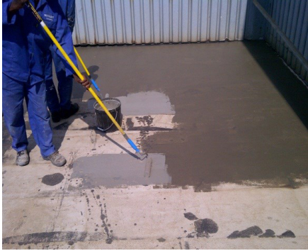
Photo 1: Flat roofing application
