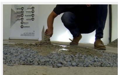
Fig 06: Trolling in LEVELiTe. Bulk up coat.
