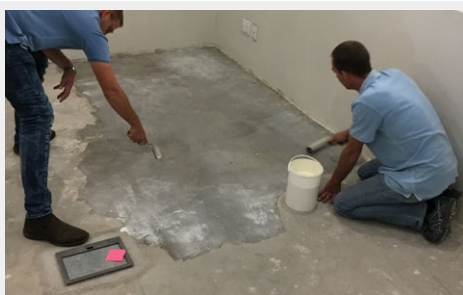
Fig 01: VAPORiTe+PLUS first coat
